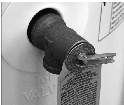
Figure 25 - Temperature and Pressure Relief Valve
