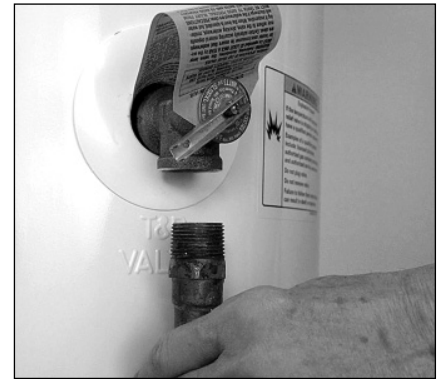
Figure 21 - Removing the T&P Relief Valve discharge pipe.
