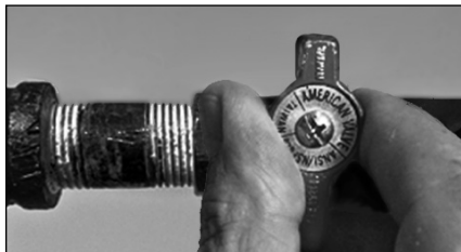
Figure 46 - Gas valve in “off” position.
