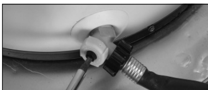
Figure 40 - Draining the water heater.
